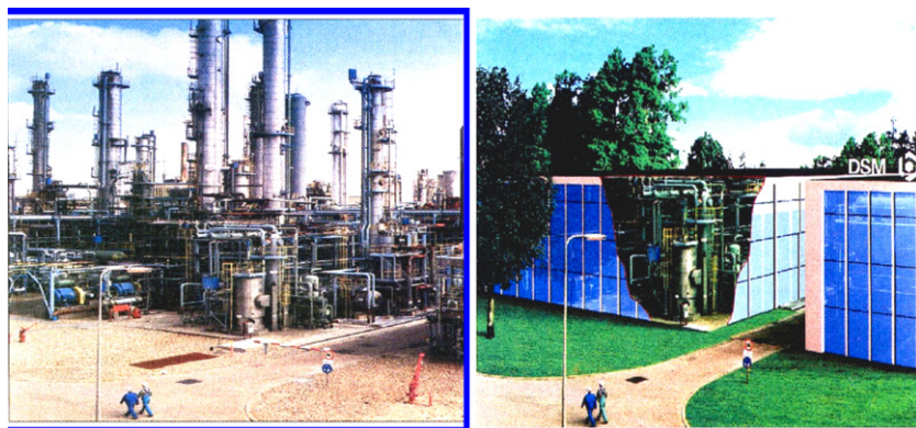
Fig. 2. One vision of how a future plant employing process intensification may look (right) vs. a conventional plant (left) [57].
